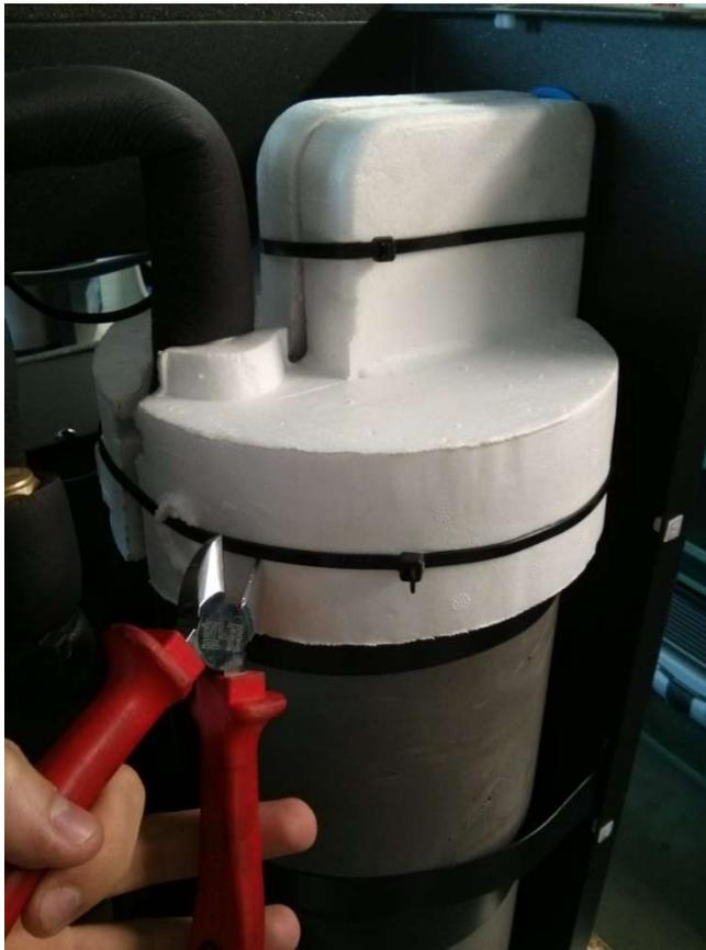
*Remove the insulation cutting the two black clamps using the tongs.*
